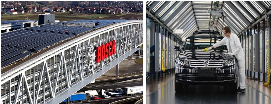
Figure 12. The new research campus in Renningen is to become the new hub of the Bosch Group's global research and advance engineering activities. The construction costs of the new campus was around 160 million Euros. Volkswagen (VW) is the single biggest industrial spender on R&D worldwide with US$17 billion on R&D in 2014. Second enterprise was Intel (USA) with US$13.6 billion for R&D.
